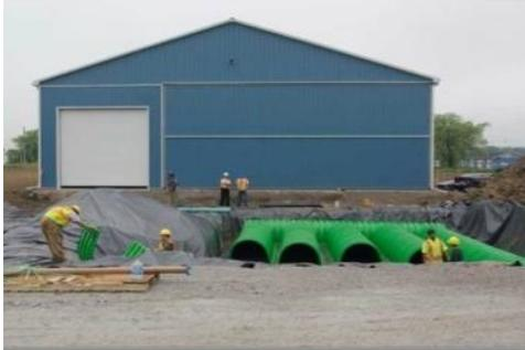
**Soakaways, infiltration trenches and chambers** and can be used to reduce runoff volume and maintain or enhance recharge. Most surface areas can be directed to infiltration practices without pre-treatment. Roads and parking lots should be provided with pre-treatment devices to prevent clogging, extend their lifecycle, and protect groundwater quality.
