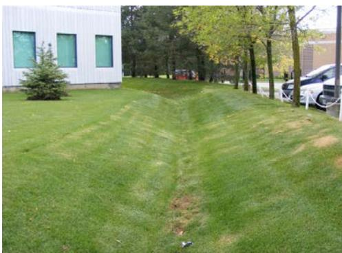
**Enhanced grass swales** are vegetated open channels designed to convey, treat and attenuate stormwater runoff (also referred to as enhanced vegetated swales). Check dams and vegetation in the swale slows the water to allow sedimentation, filtration through the root zone and soil matrix, evapotranspiration, and infiltration into the underlying native soil. Simple grass
