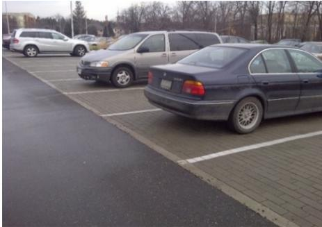
**Partial** permeable pavement parking surface has permeable pavement that is strategically constructed within the parking stall areas only and the central drive-lanes remain as conventional asphalt. In this manner, the permeable pavement systems can accept runoff from impervious areas (i.e. drive lanes).
