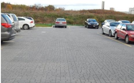
**Full** permeable pavement parking surface has permeable pavement for drive lanes and parking stalls.
