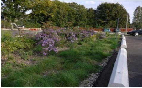
As a stormwater filtration and infiltration practice, **bioretention** temporarily stores, treats and infiltrates runoff. The primary component of the practice is the bioretention soil media. This component is comprised of a specific ratio of sand, fines and organic material. Another important element of bioretention practices is vegetation, which can be either grass or a more elaborate planting arrangement such as an ornamental garden.
