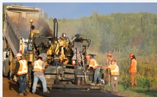
Figure 3. FPIInnovations – Lignin Modified Asphalt Test Sections
