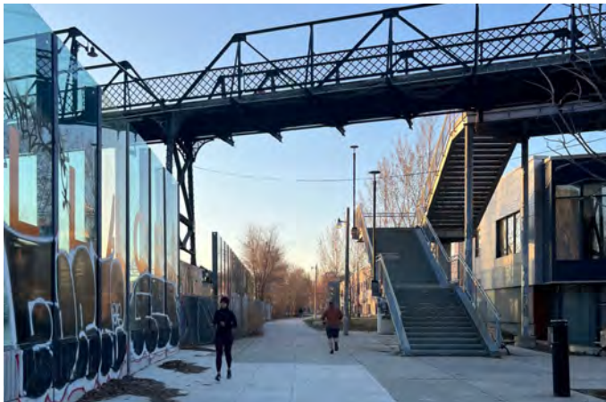
Figure BL Bike Ramps Integrated into Stairs
