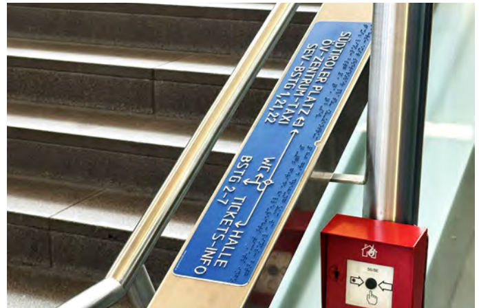
Figure AR Braille at the Bottom of Stair Railings
