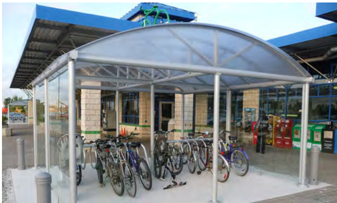
Figure BP Bike Parking at GO Station
