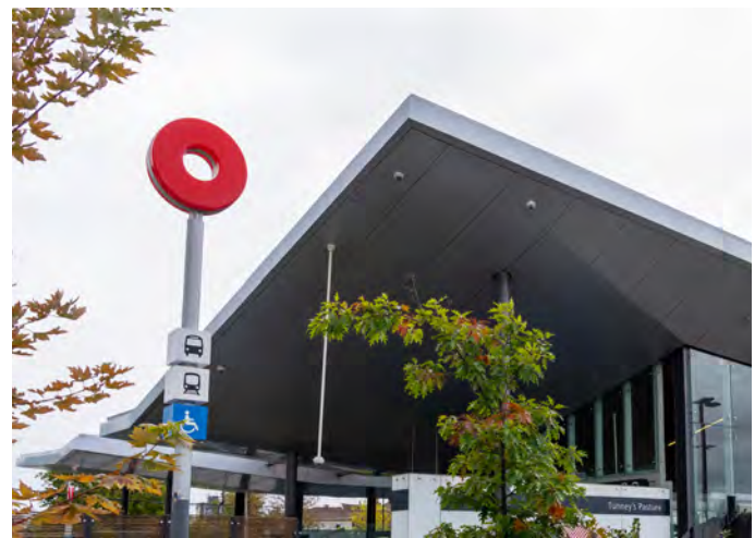
Figure AP Overhead Canopy Structure Provides Sense of Entrance and Weather Protection
