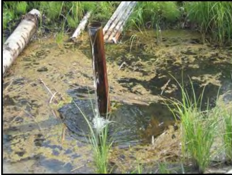
Photo 11: Drill hole with casing producing water, before being sealed.
