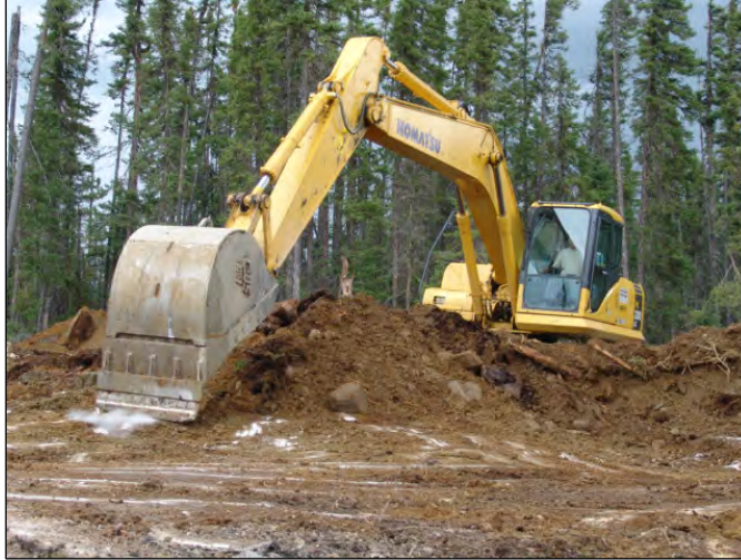
Photo 3: Backhoe being used to strip overburden.
