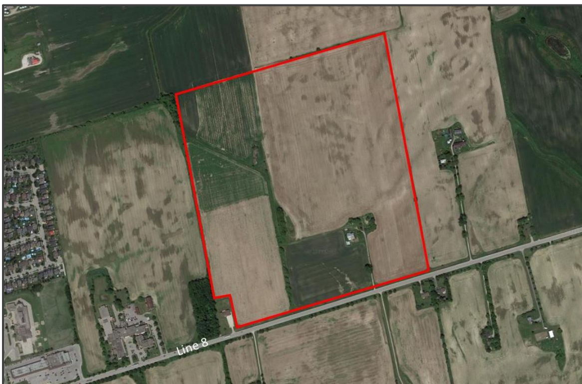
Figure 1: Air Photo of the Subject Lands
