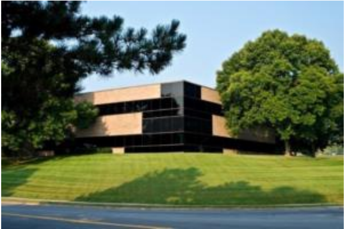
Case study site: Office building – Latham, NY
